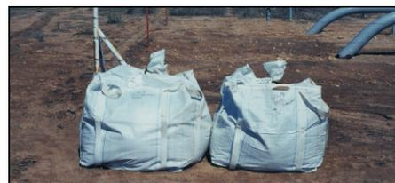
*Excavated soil placed into soil bags awaiting characterization for disposal.*
