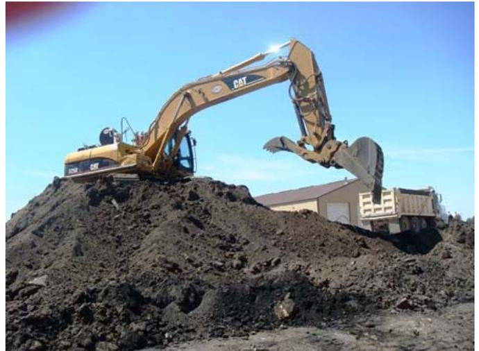
*Excavating the fill material used to build the parking lot.*
