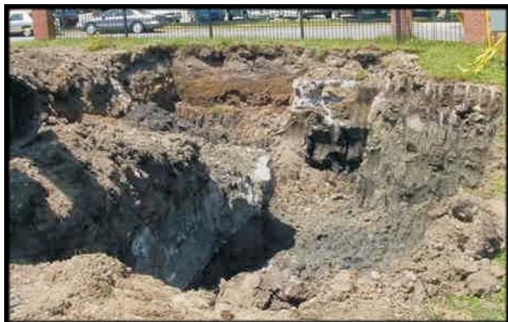
Contaminated soil excavation and removal.
