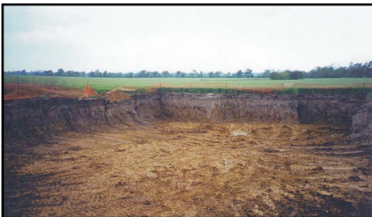
Completed excavation, May 1999
