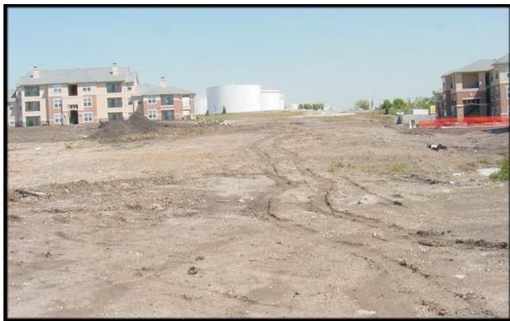
Contaminated soil excavation and removal.
