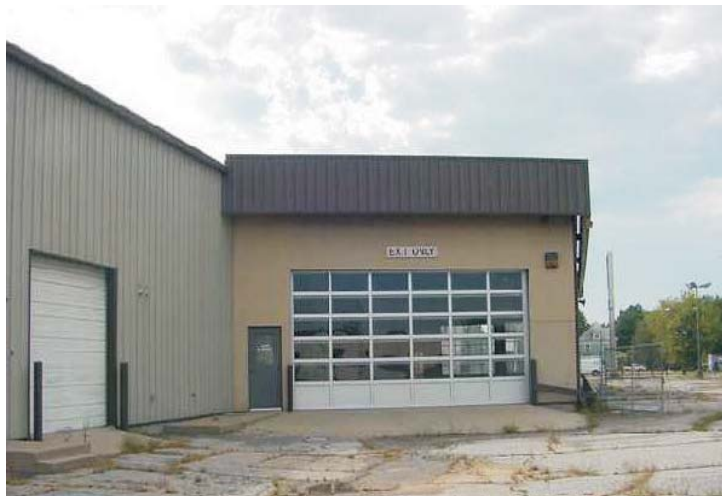
Former Car Dealership and Maintenance Facility on Site
