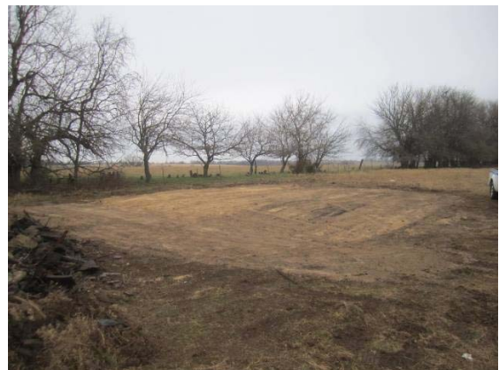
Backfilling and grading restored the site's natural condition..
