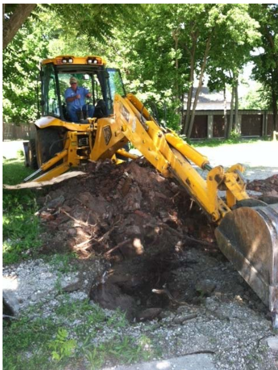
Excavating lead-contaminated fill material.
