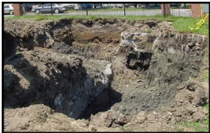
Contaminated soil excavation and removal.
