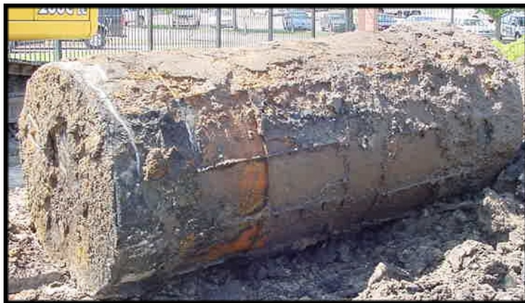
Excavated drum before taken off-site
