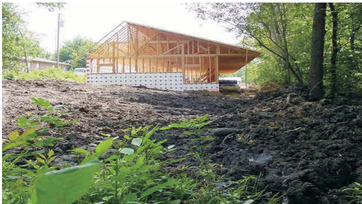
Redevelopment under construction
