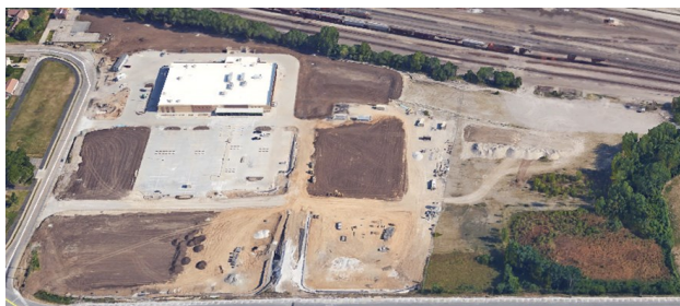
Aerial of site during construction; Walmart almost complete.
